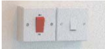
The dual box will accept two single switch plates. Neater than using two separate boxes and more convenient when bringing cable through a wall
