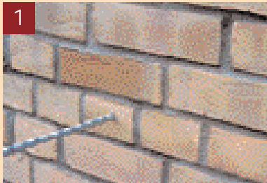
1 Drill a 10mm hole through your house wall at a convenient point
