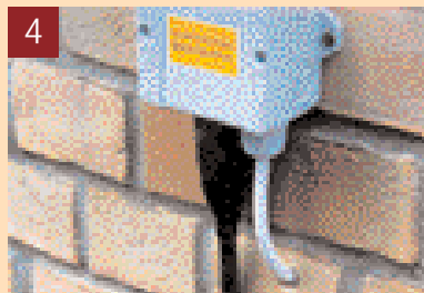
4 The unit must be connected to the power supply with an RCD
