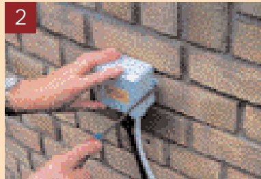
2 The exterior waterproof junction box is fitted to the wall
