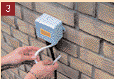
3 The box is ready wired to armoured cable. Feed other cable into the wall
