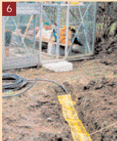
6 Warning tape is laid over the top as an extra safety device
