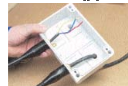
The thinner wires on the left are switch wires and are all phase conductors and therefore do not need flagging
