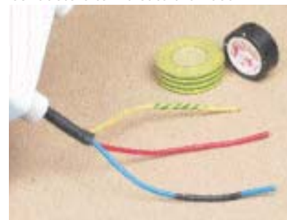
Using insulation tape to 'flag' the conductors to indicate their use
