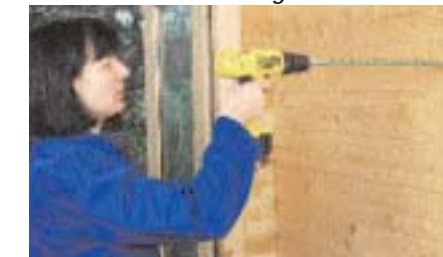
A long drill bit will help keep those holes straight and prevent the conduit from binding
