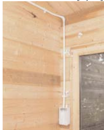
Run all the conduit before installing any wiring
