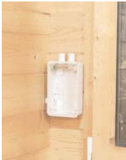
The consumer unit case is installed first
