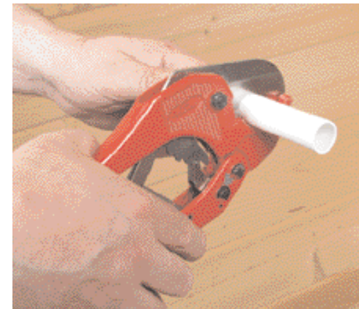
Cutting the conduit with pipe shears makes a neat job
