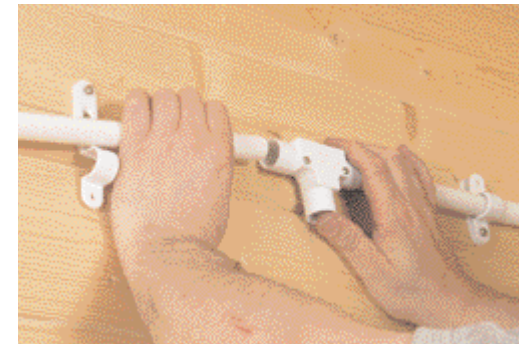
Access plates should always face outwards
