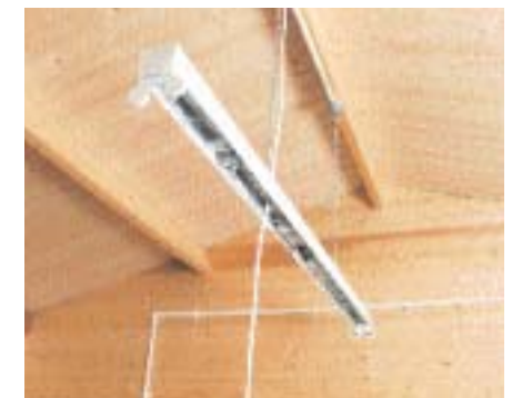
The lights are hung on Jack chain from hooked conduit box lids. These are fixed to the boxes with brass screws. The flex is run down the chain and into the fittings
