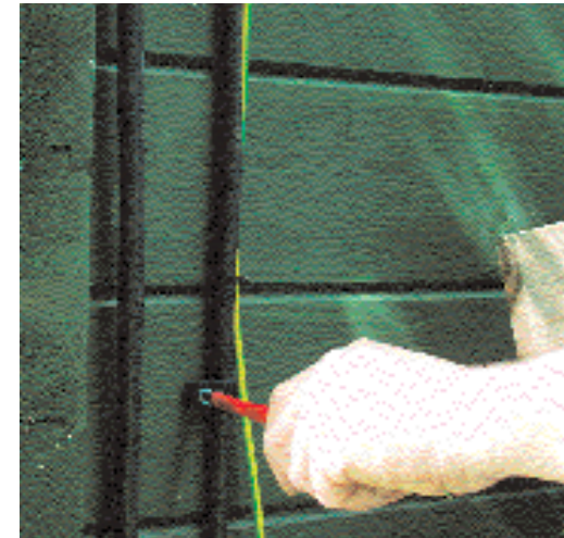
Once the armoured cables have been fitted to the box they can be fixed to the outside wall with cable clips. The cable connecting the earth pole to the block is held in place with cable ties
