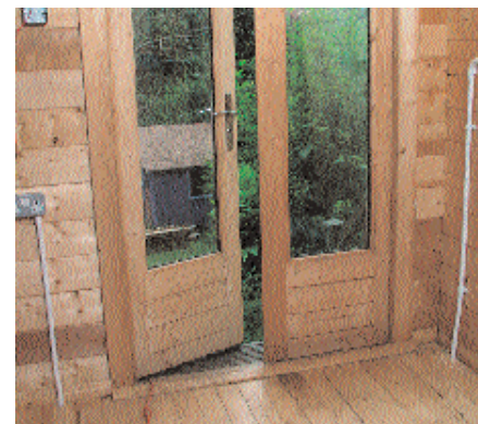
The ring circuit is completed by running the conduit under the floor. This avoids lots of unsightly conduit bridging the door opening
